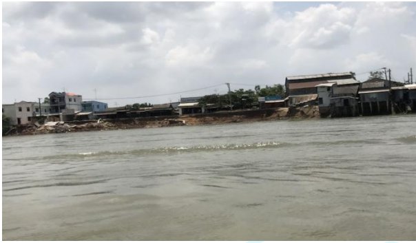
Photo: Scene of landslide aftermaths in Block 12, My Hoi hamlet, My Hoi commune, Cho Moi district in April 2017
