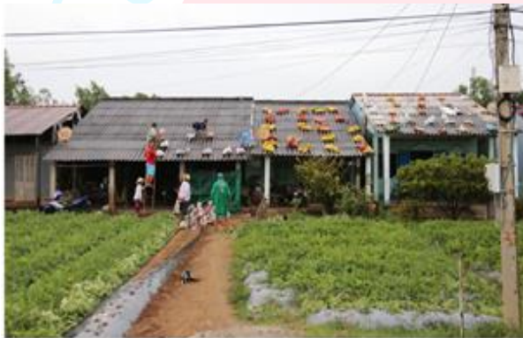
Photo: People in Tran De district (Soc Trang) braced their houses to actively respond to Typhoon No. 16.
