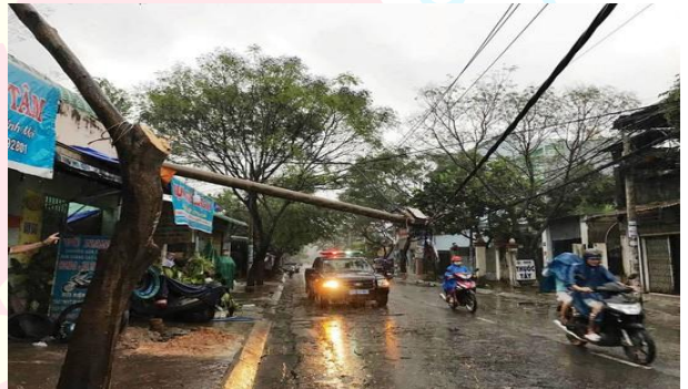
Photo: Damages caused by Typhoon No.14 in Ho Chi Minh City
